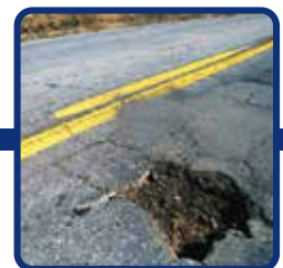
POTHoles/DAMAGED PAVEMENT
