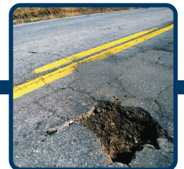
POTHoles/DAMAGED PAVEMENT
