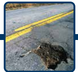
POTHoles/DAMAGED PAVEMENT
